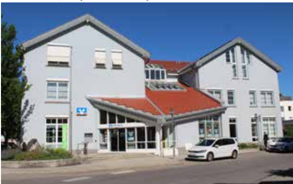
Abb.78: VR-Bank, Ruderatshofefer Straße 1
